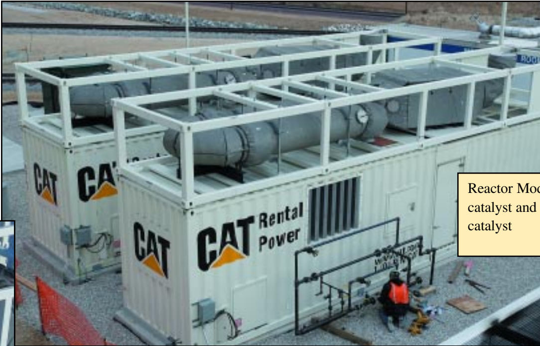
SCR System shown mounted on Cat® G3516 Power Module
